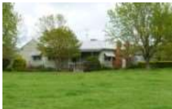
The original home of Rene and Norm Trewella where they raised their children Ron and Cecily
